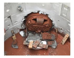
At intervals, large drive and reception shafts (for the tunnelling machine) were constructed, again overseen by archaeologists. The drain was also tunnelled several metres beneath the medieval city wall so that this was not disturbed.
